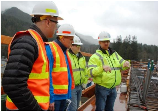
Tacoma Water Project Engineers, Jason Moline (right) and Gary Fox (center right), on the deck of the new flocculation basins with Secretary of Health John Wiesman (center left) and Deputy Secretary Dennis Worsham (left) during a January 2014 site visit.
