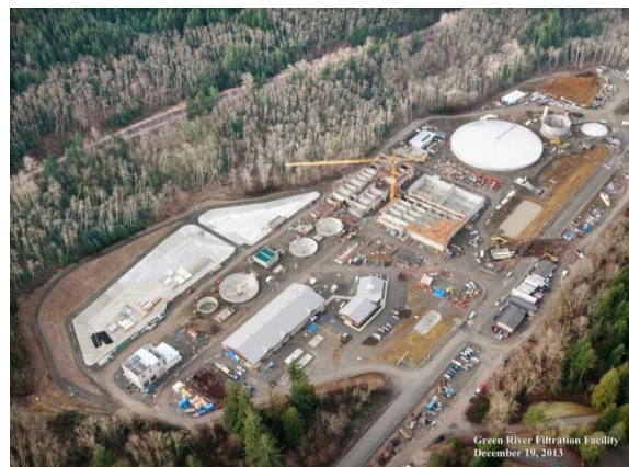
The Green River Filtration Facility covers about 25 acres.
