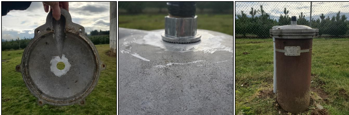
Figure 13: Top and bottom surface ground smooth with \frac{1}{2} " watertight hub and nipple installed ready for the Ranger
