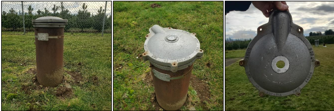
Figure 12: Aluminum Well Cap with \frac{3}{4} " hole drilled in center for watertight hub.
