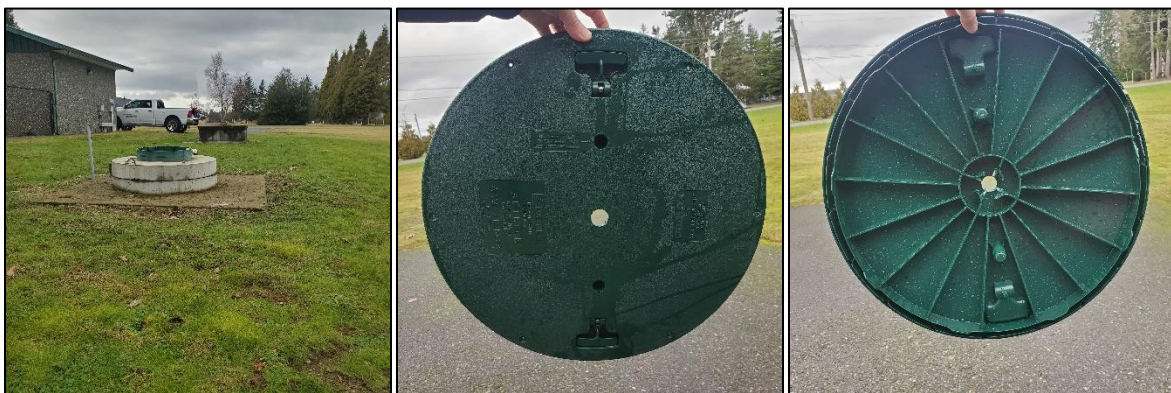
Figure 14: 36" Cement Cap with imbedded PVC Hatch with \frac{1}{2} " hole drilled in the center for watertight hub
