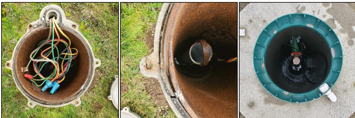
Figure 18: Common Well Obstructions
