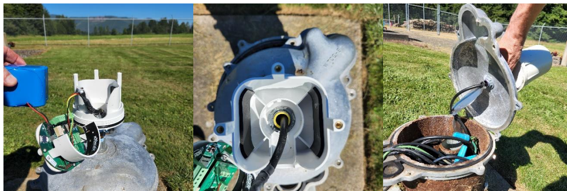
Figure 21: Transducer Wire Install to Ranger
